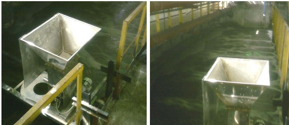
Figure 4 Zeolite dosing by automatic tenzometric dosing system at Golden Sands WWTP
